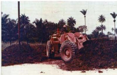
Fig 39c Front-end loader turning
