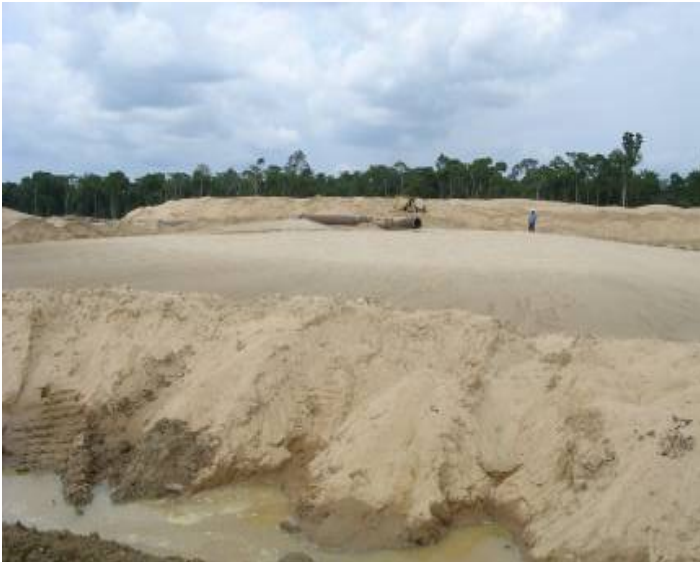
Fig 4.0: Dredging and Sand filling
