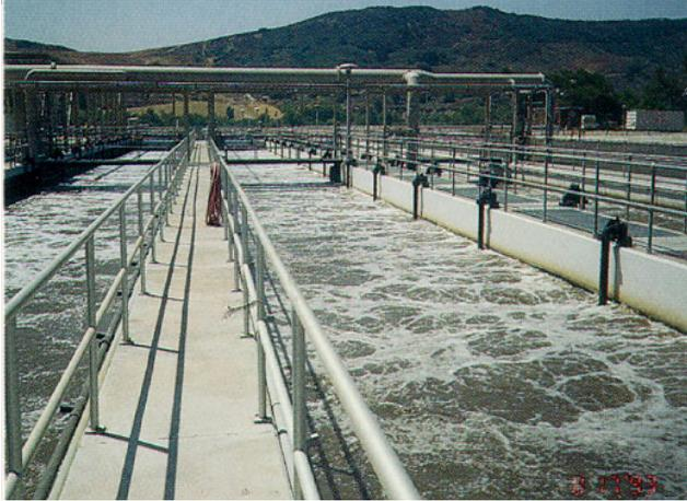
**Fig 23 Activated sludge**
